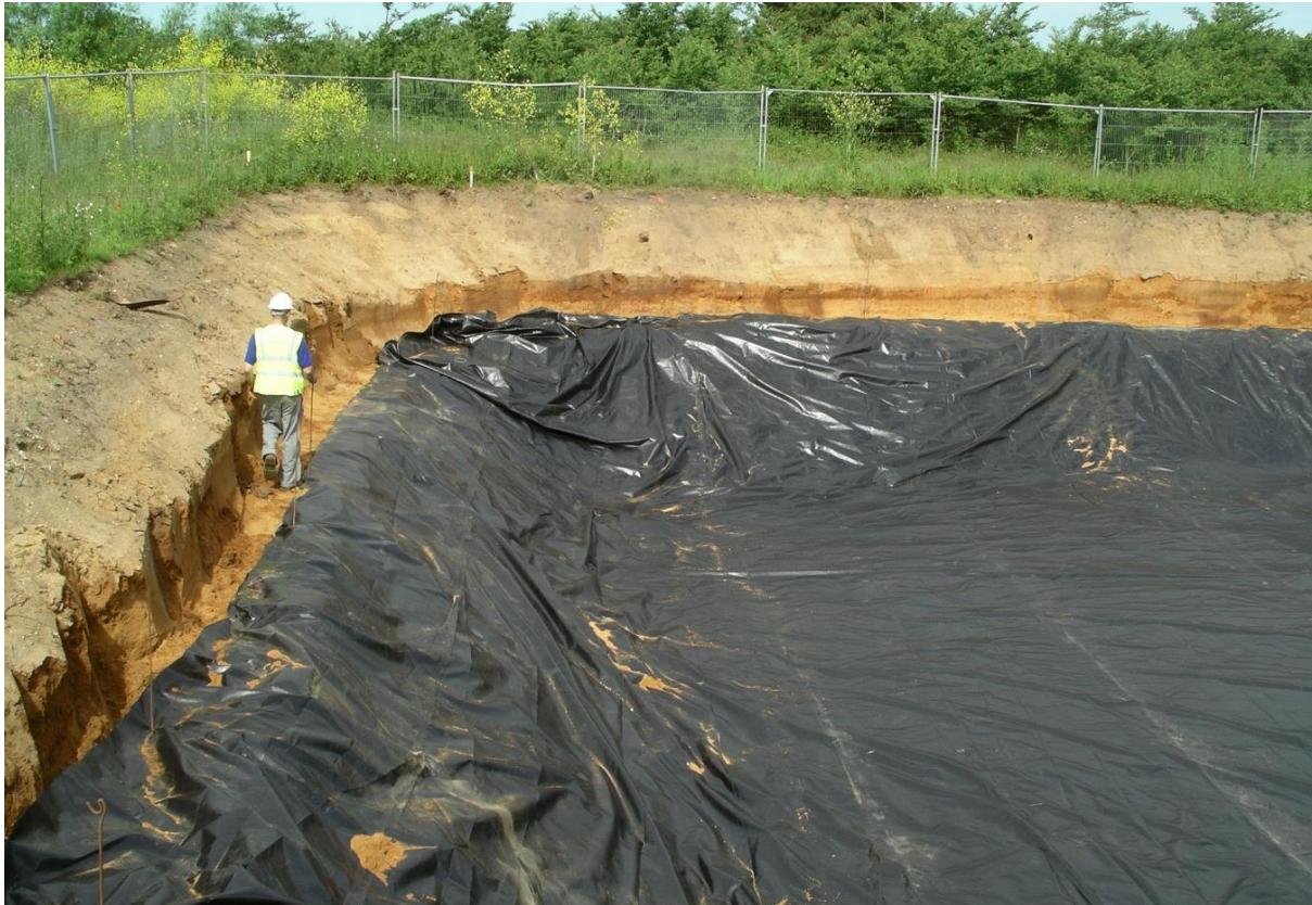
Installing the cell liner.
