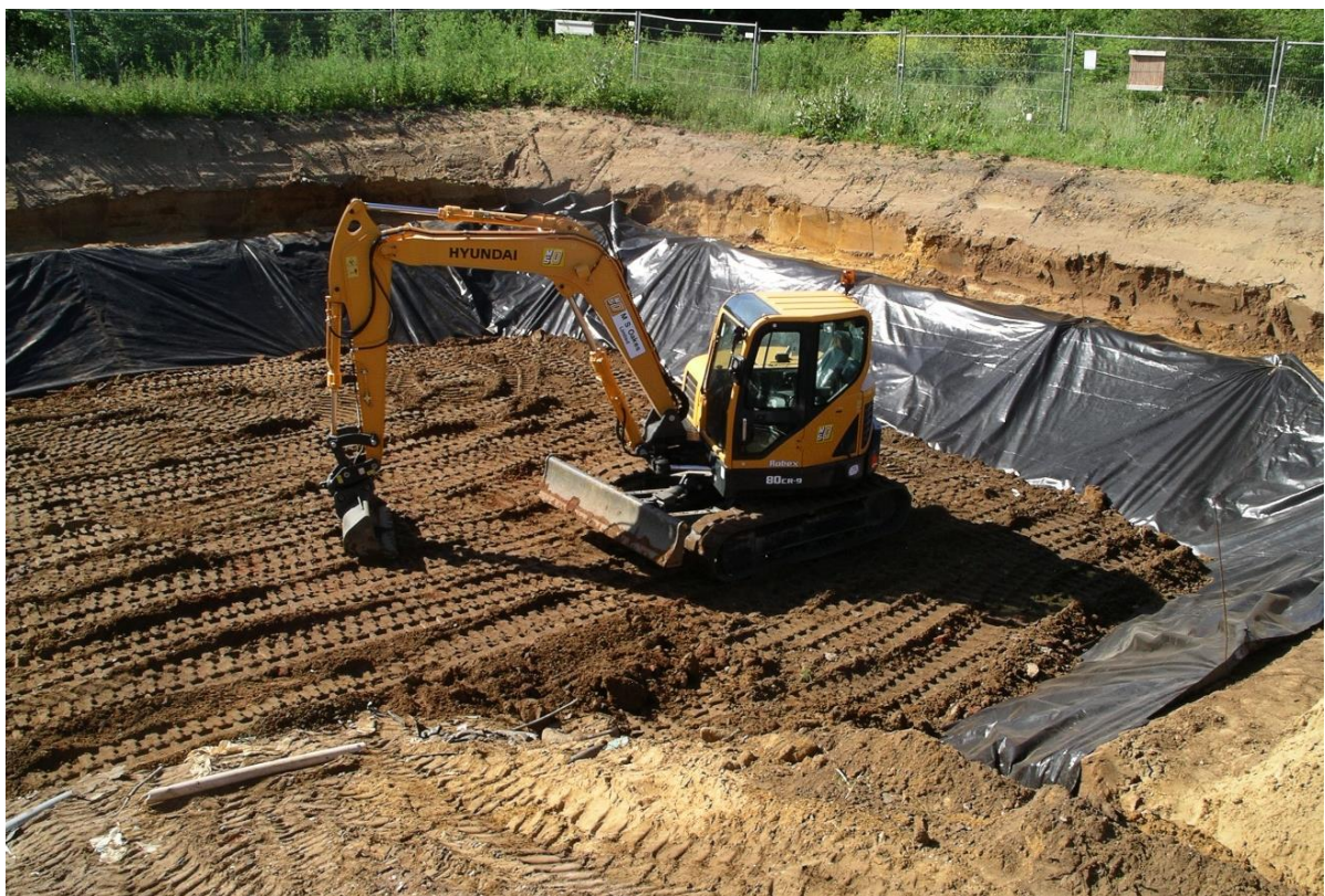
Filling the cell with the excavated Japanese knotweed soils.
