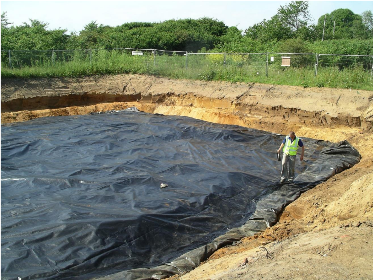
Sealing the cell burial.
